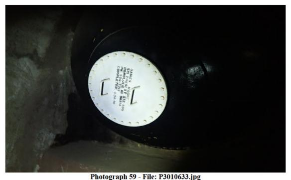
Tank 10 manhole cover and maintenance door. Note that the bolts do not have washers. The EPA Inspection Team did not observe a gasket between the outer plate and manway hole.
