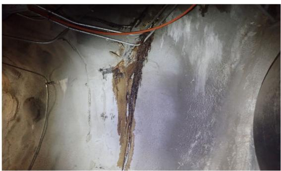
Photograph 71 - File: P3010645.jpg Staining on wall near Tank 15.
