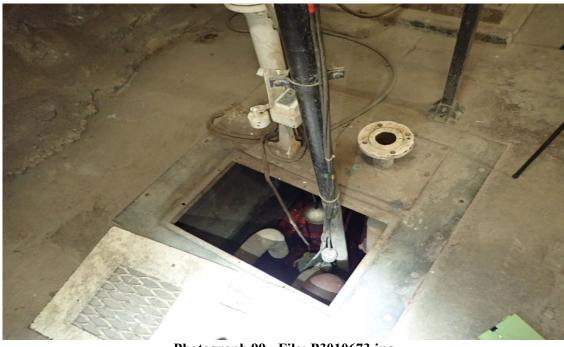
**Photograph 99 - File: P3010673.jpg**Zone 7 Fuel Oil Reclamation Sump in the Lower Access Tunnel.
