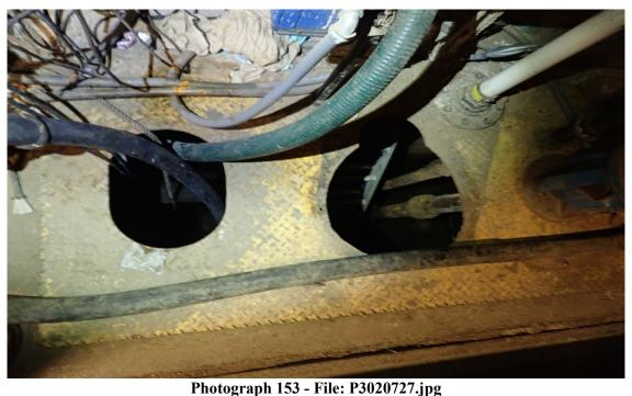
Adi groundwater sump. Facility personnel explained that spilled fuel had discharged into this sump, which is located approximately (b) (3) (A) from the point where fuel was released.
