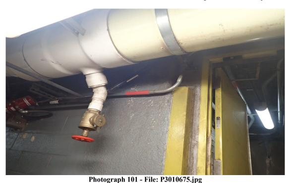
Low point on AFFF line in the Lower Access Tunnel. Portions of the AFFF line are metal and PVC. This image shows the PVC portion.
