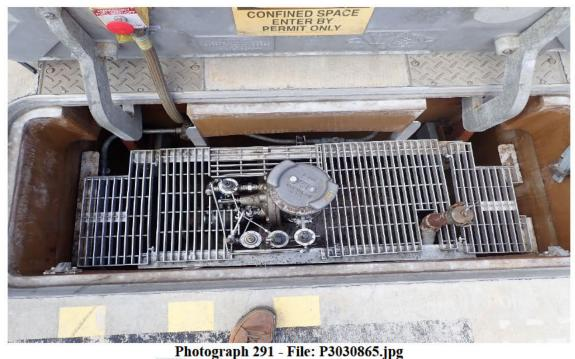
Diamond Head hydrant pit with minor amount of accumulated fluid with a odor of petroleum.
