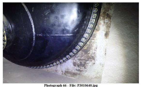
Tank 12 manhole cover and maintenance door. Note that the bolts do not have washers. The EPA Inspection Team did not observe a gasket between the outer plate and manway hole.
