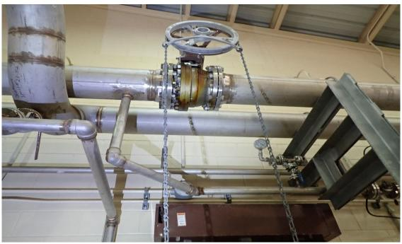
Photograph 288 - File: P3030862.jpg Leaking valve in the Ewa Pump House.
