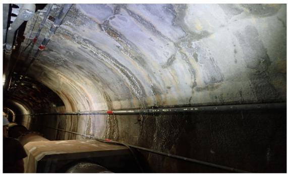
Photograph 178 - File: P3020752.jpg Salt or other crystalline deposits on the wall in the Lower Access Tunnel.
