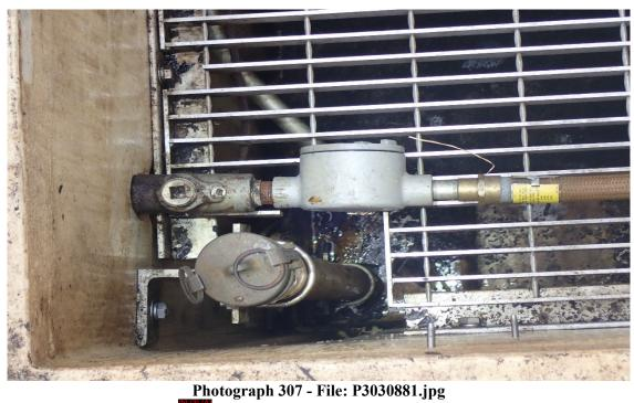
Hydrant Pit with accumulated liquid.
