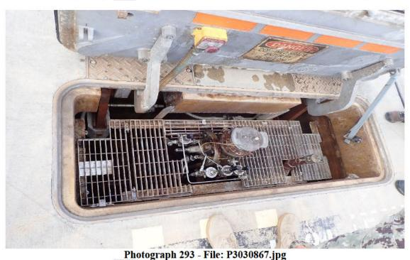
Diamond Head hydrant pit with minor amount of accumulated fluid with odor of petroleum.
