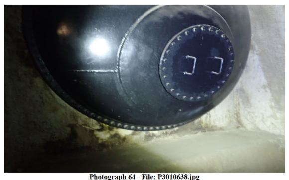
Tank 11 manhole cover and maintenance door. Note that the bolts do not have washers. The EPA Inspection Team did not observe a gasket between the outer plate and manway hole.
