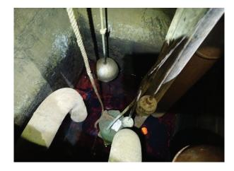
Figure 2: Zone 7 Sump for Fuel Oil Reclamation
