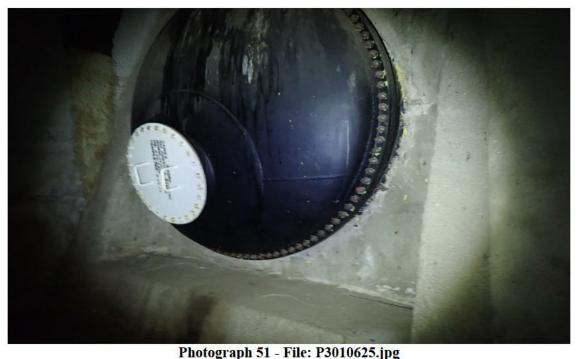
Tank 8 manhole cover and maintenance door. Note that the bolts do not have washers. The EPA Inspection Team did not observe a gasket between the outer plate and manway hole.
