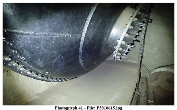
Tank 2 manhole cover and maintenance door. Note that the bolts do not have washers. The EPA Inspection Team did not observe a gasket between the outer plate and manway hole.
