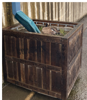
A Grattix box after installation at the project site.
