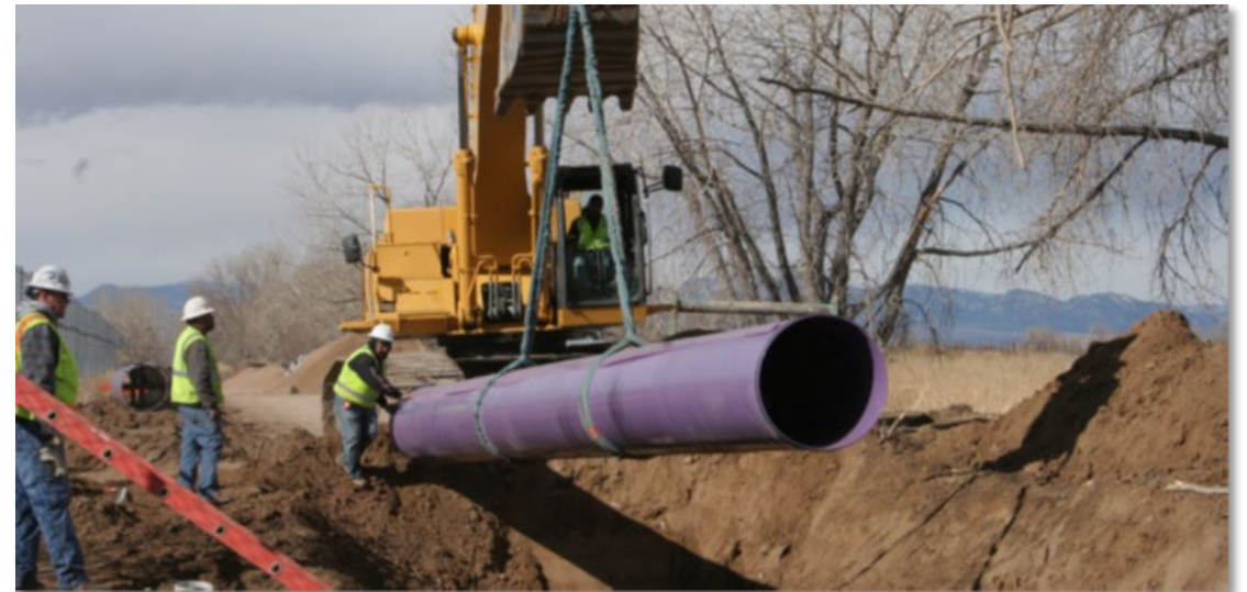
Denver Water contractors install a purple pipe used to deliver recycled water in northeast Denver, Colorado
