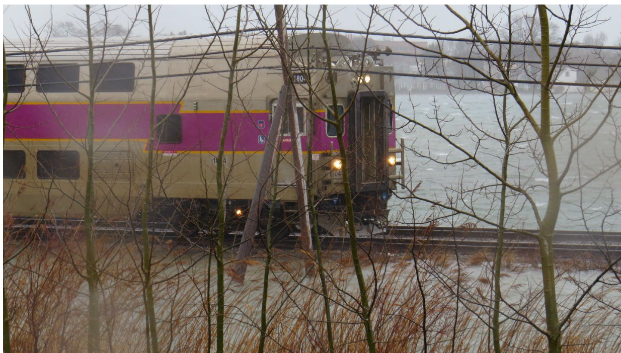
Figure 32. Photograph taken March 3, 2018, shows tidal water levels approaching the top of the railroad embankment at Rumney Marsh. Photo credit, Geoffrey Wilson, Northeast Wetland Restoration.
