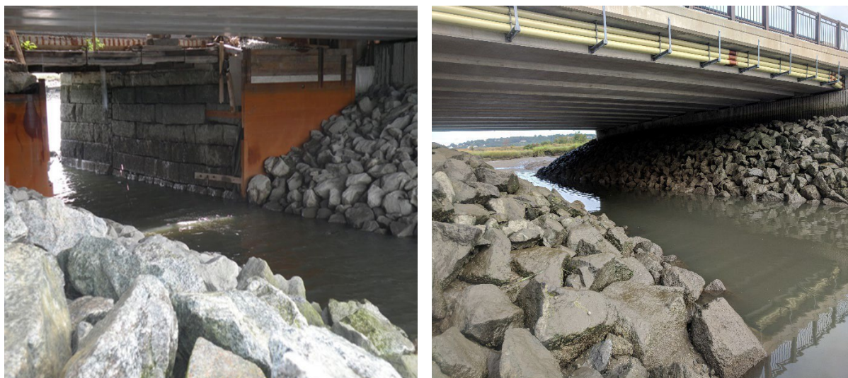
Figure 9. During and after construction photographs of the East Branch Pines River bridge S-5-3 crossing show how the vertical walls of the former bridge were changed to a riprap slope, which increased channel conveyance. Photo credit Ed Reiner.
