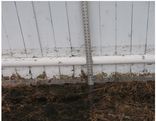
Figure C-26. January 30, 2018 high tide debris 18-inches high estimated elevation 7.1 feet NAVD88. Photo credit Fae Saulenas.
