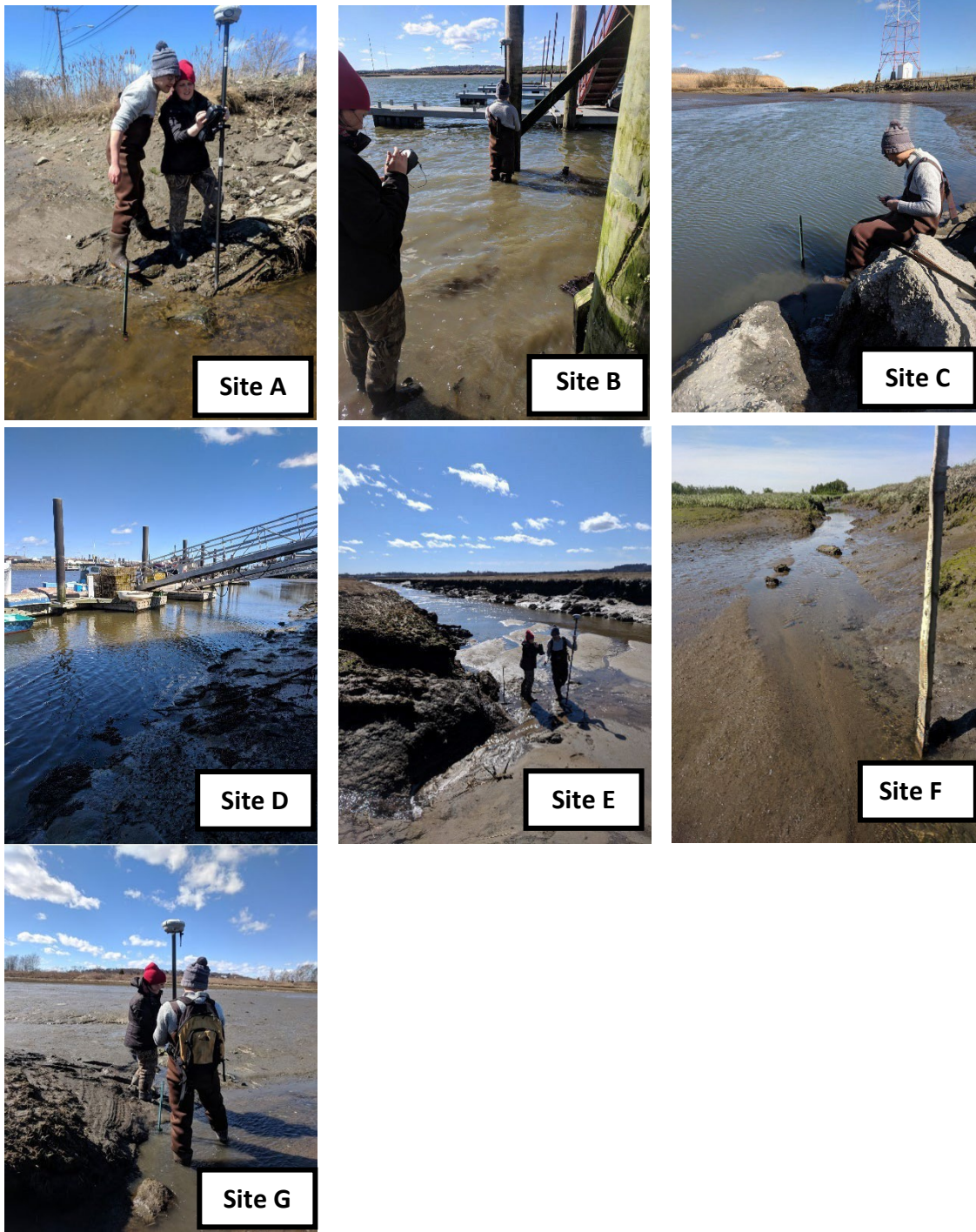
Figure 17. Photographs of the pressure transducer installations at sites A – Ballard Street, B – Lower Pines River, C – Upstream Railroad, D – Saugus River, E – Upstream I-95, F – East Saugus, and G – Upstream 107. Photo credit Ed Reiner.
