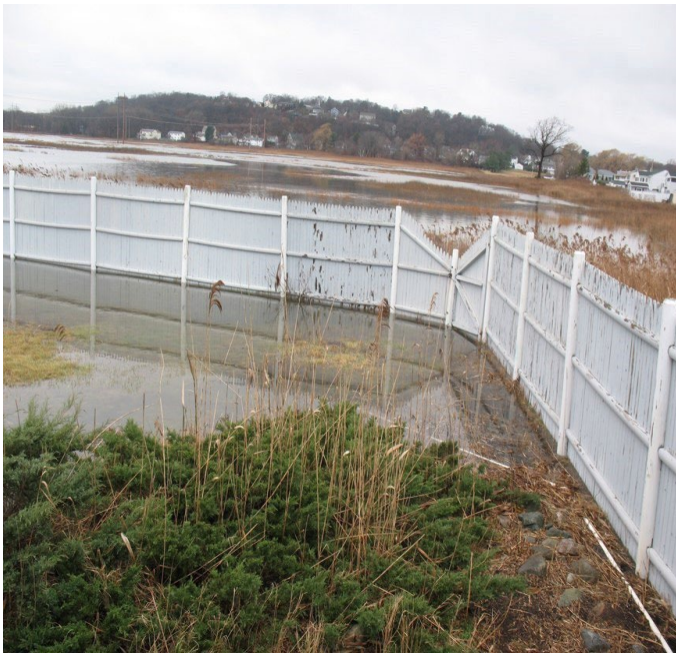
Figure C-16. November 25, 2018, high water level estimated at elevation 6.4 feet NAVD88. Photo credit Fae Saulenas.
