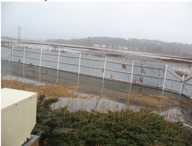
Figure C-12. February 7, 2020, high water estimated at elevation 6.4 feet NAVD88. Photo credit Fae Saulenas.
