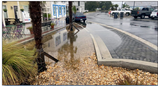
Figure 2. A bioretention system at “Market on Square” reaches capacity and overflows onto permeable pavement (St. Marys Street).
