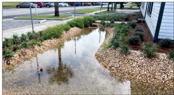
Figure 3. A full bioretention practice near City Hall (Osborne Street) with monitoring wells in the foreground.
