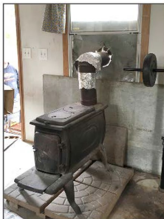
An example potbelly stove installed in a household with improper venting and clearances (left), and the scorching on the wall that resulted (right). The authors noted that the flue was completely clogged with creosote upon removal (Stove Stories, n.d.)
