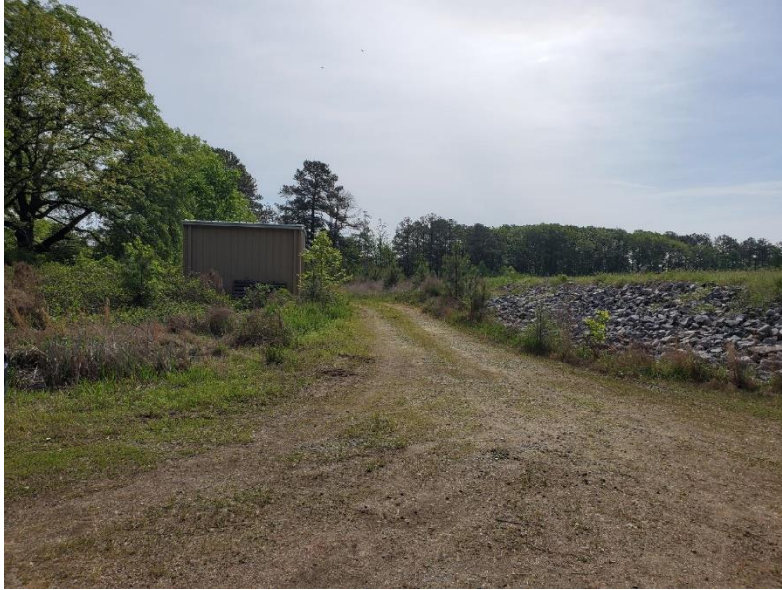
Facing East. Storage shed includes PPE, various equipment, and some hazardous waste stored according to permit.
