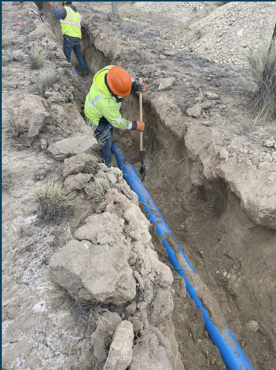
Workers installing new water main.
