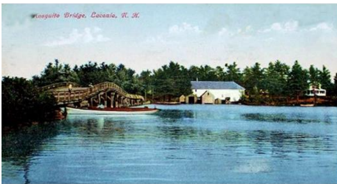
Mosquito Bridge, Laconia.
