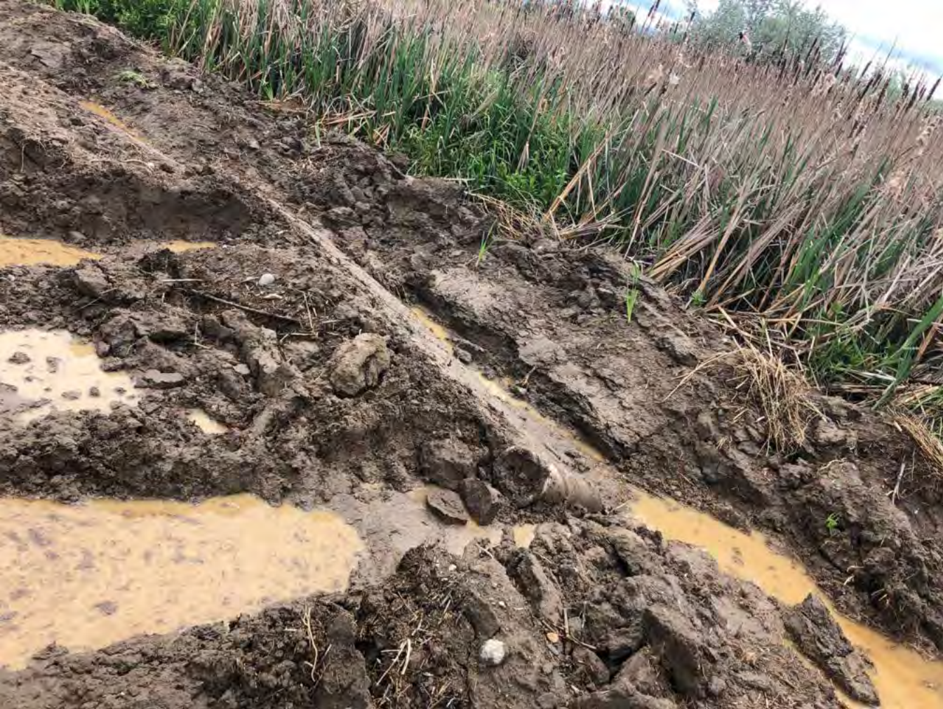
Photograph taken by Inspector Montague on May 21, 2019 facing 113 degrees southeast shows where field lateral that borders facility meets ditch along the north and northwest side of Owyhee Dairy. Bank has been compromised and runoff from corrals is able to commingle with ditch water.
