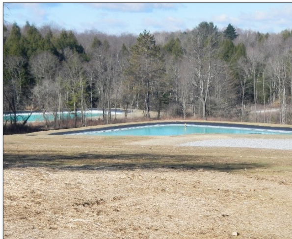
Figure 2. Fall Brook AMD passive treatment system.
