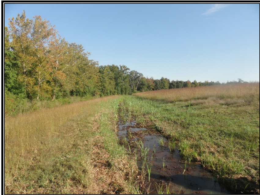
Photograph No. 14: Northerly view of ponding in a stormwater swale along the northwesterly margin of SWMU 17, a coal ash landfill. The ponding was addressed as non-conformance with Solid Waste Post-Closure Permit SW-09/01.
