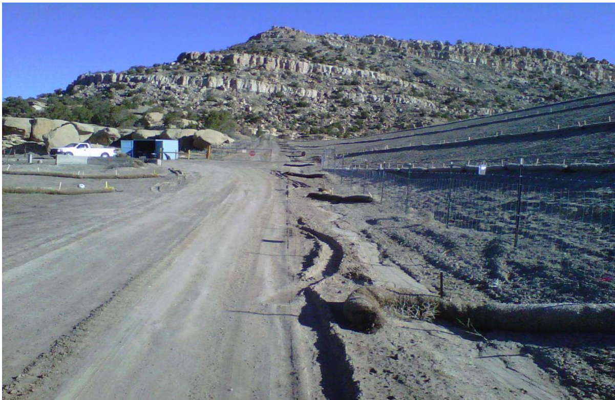
Plate 3.3-3 West Slope of Waste Rock Pile with Erosion Controls
