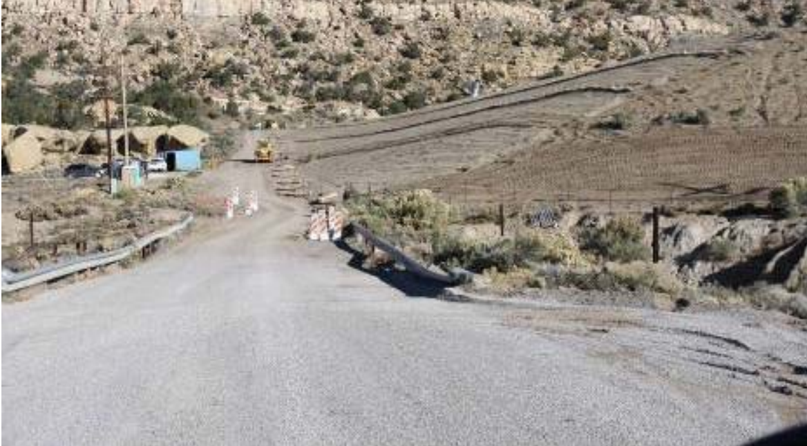
Plate 3.3-2 View of Entrance Ramp Showing Road and Waste Rock Pile Mitigation
