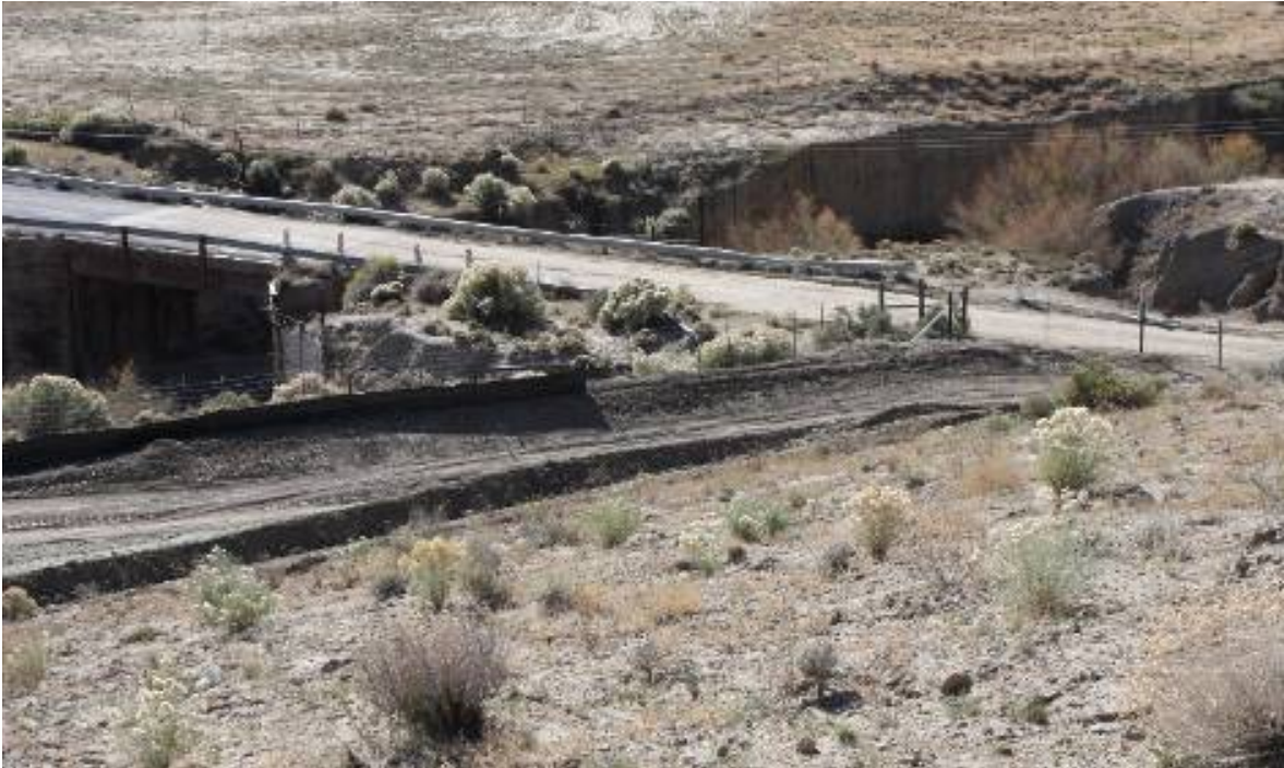
Plate 3.3-4 Berm Storm Water Control at South End of Waste Rock Pile
