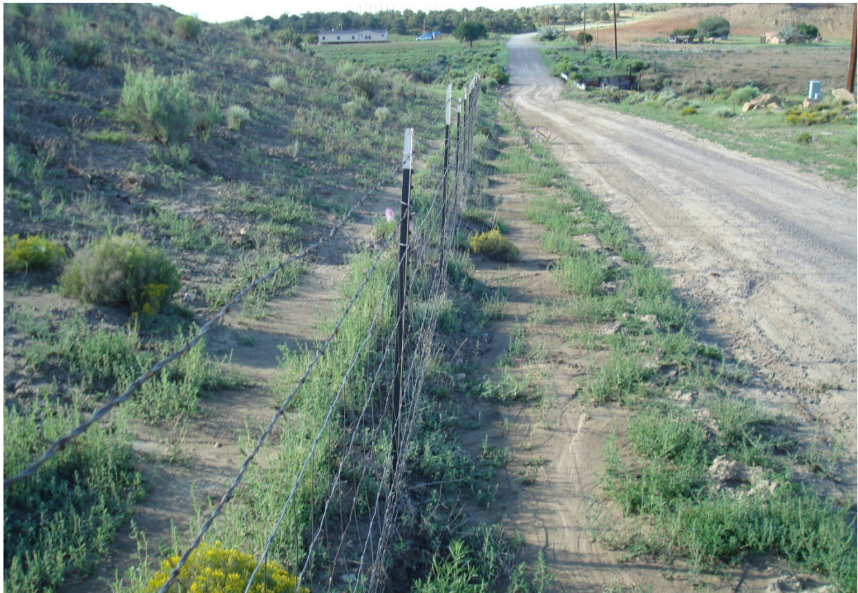
Plate 3.3-1 West Slope of Waste Rock Pile Prior to Mitigation
