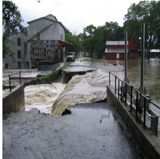
Failure of Hearn's Pond dam near Seaford in August 2001.
