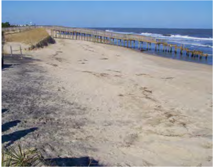
Storm Related Coastal Erosion in Bethany Beach Delaware: Following a severe extratropical coastal storm in November 2009. The pre-storm profile of the dune is evidenced by the wooden dune crossover profile. There appears to be over 50 feet of horizontal dune loss and significant beach erosion at this location. (DNREC Photo)
