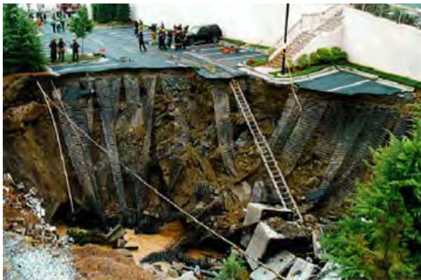
Collapses, such as the sudden formation of sinkholes, may destroy buildings, roads, and utilities. (Photo: Bettmann)
