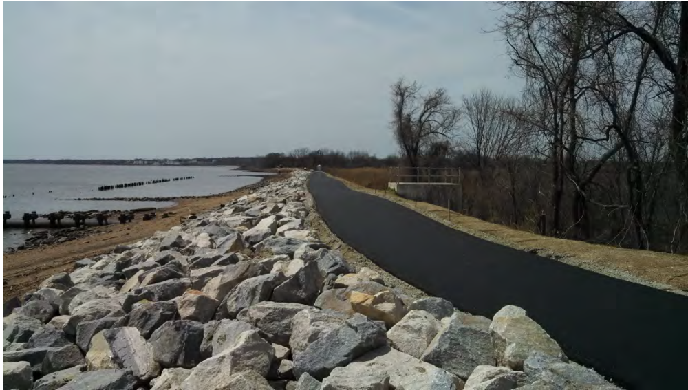
Gambacorta Dike in New Castle, DE
