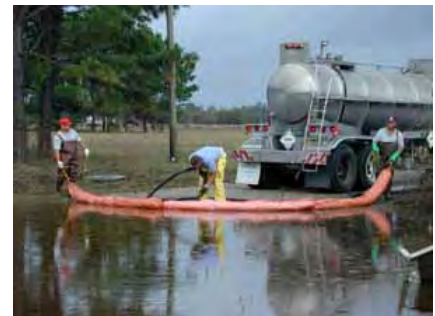
Propane tanks, gasoline, oil and other hazardous materials and debris in Princeville, North Carolina were cleaned up by Environmental Protection Agency crews following Hurricane Floyd in September 1999. The town remained off limits to residents for some time due to health-related concerns. (Photo by Dave Saville/FEMA News Photo)
