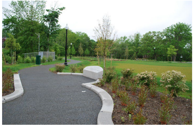
Example of permeable pavers.
