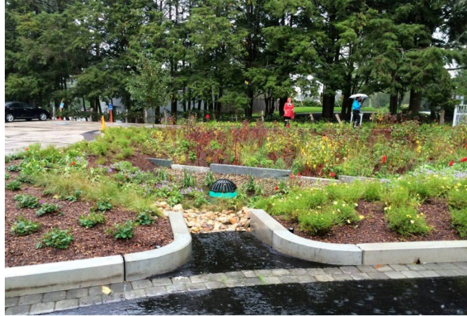
Example of bioretention system.
