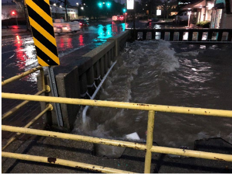
View of flooding in Gordon's Creek.
