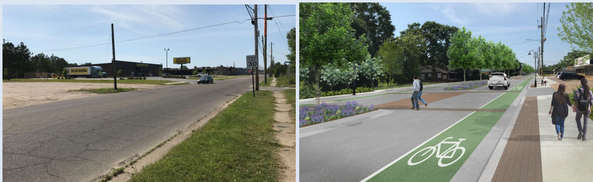
Figure 8. (Left): Current condition of Edwards Street just north of Milton Barnes Avenue, facing south.
