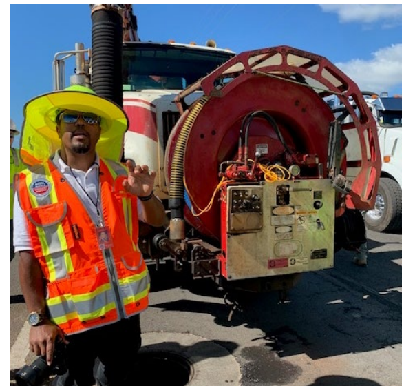
Figure 1.: EPA Wastewater Task Force Leader explains how the CCTV truck helps assess the condition of sewer lines.
