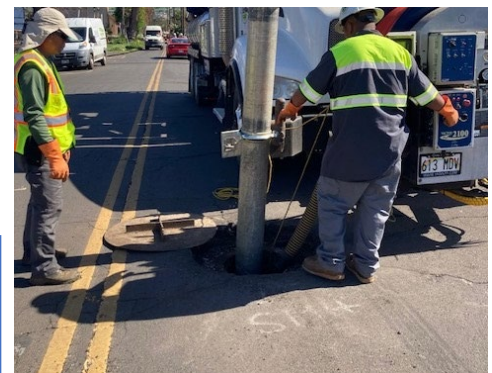
Figure 2. EPA contactors injecting water into a sewer pipe to remove any debris/blockages.
