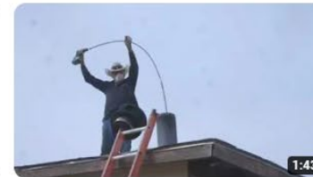
Intro To Chimney Pipe Cleaning 145 views • 2 years ago
