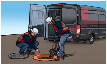
Clearing Sewer Lines: First, the work involves a crew with a jet/vacuum truck to clear the sewer lines. The crew opens two manholes within the street to gain access and pushes water at a high speed between the manholes to clear the line of debris. The debris is then vacuumed up and placed into a sealed tank.
