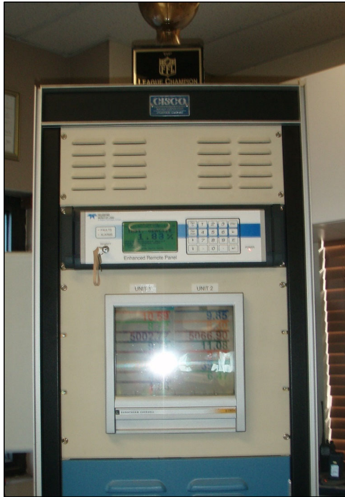
Photograph 2: View of visual display of CEMS real-time data in the facility's engineering control room.
