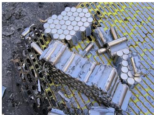
Figure 3: The intact batteries inside the apparently destroyed component.
