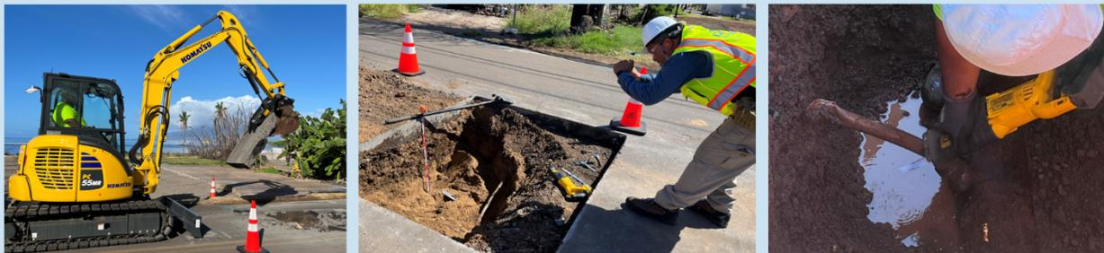
Figure 1: Prior to the start of work, crews eliminate asphalt and concrete around the excavation; an inspector inspects the excavation; a crew member cuts on a lateral line with a saw.
