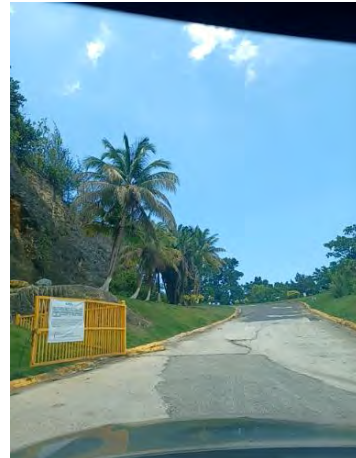
Figure 3 Inside of Gate
