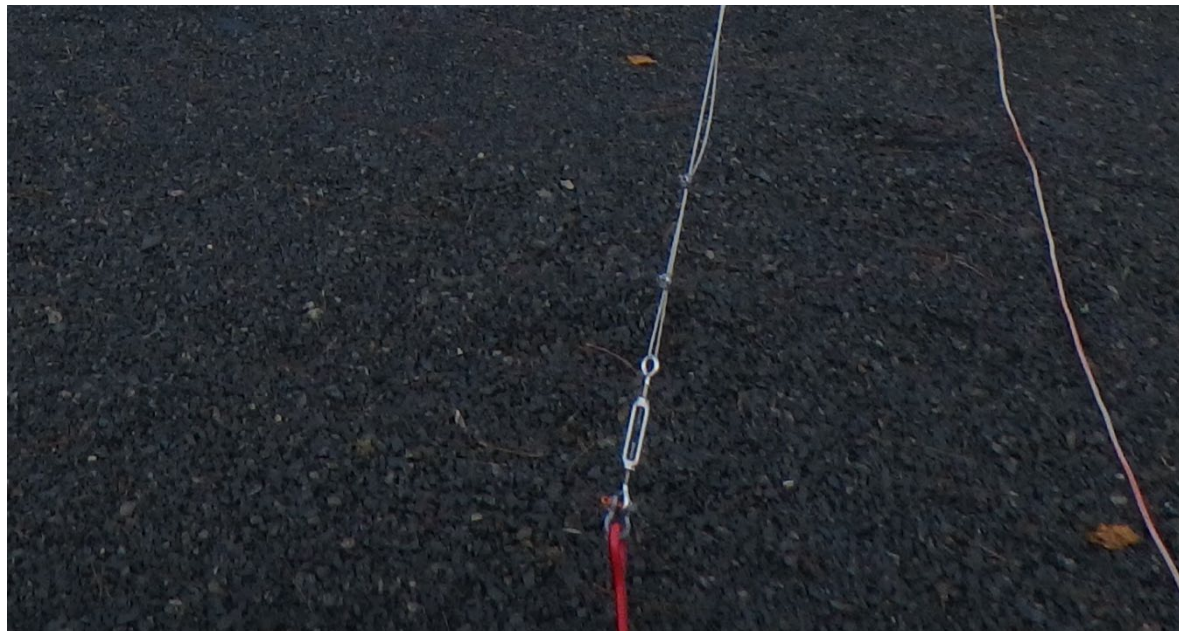
Figure 3. Guy wire attached to ground anchor
