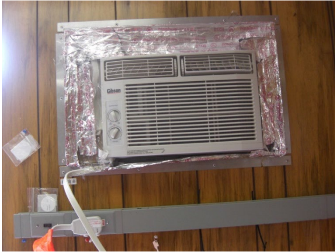
Figure 23. 120VAC Power Outlet switched by temperature control system
