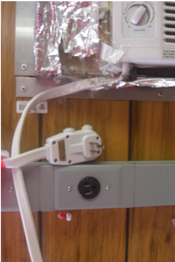
Figure 23. 120VAC Power Outlet switched by temperature control system
