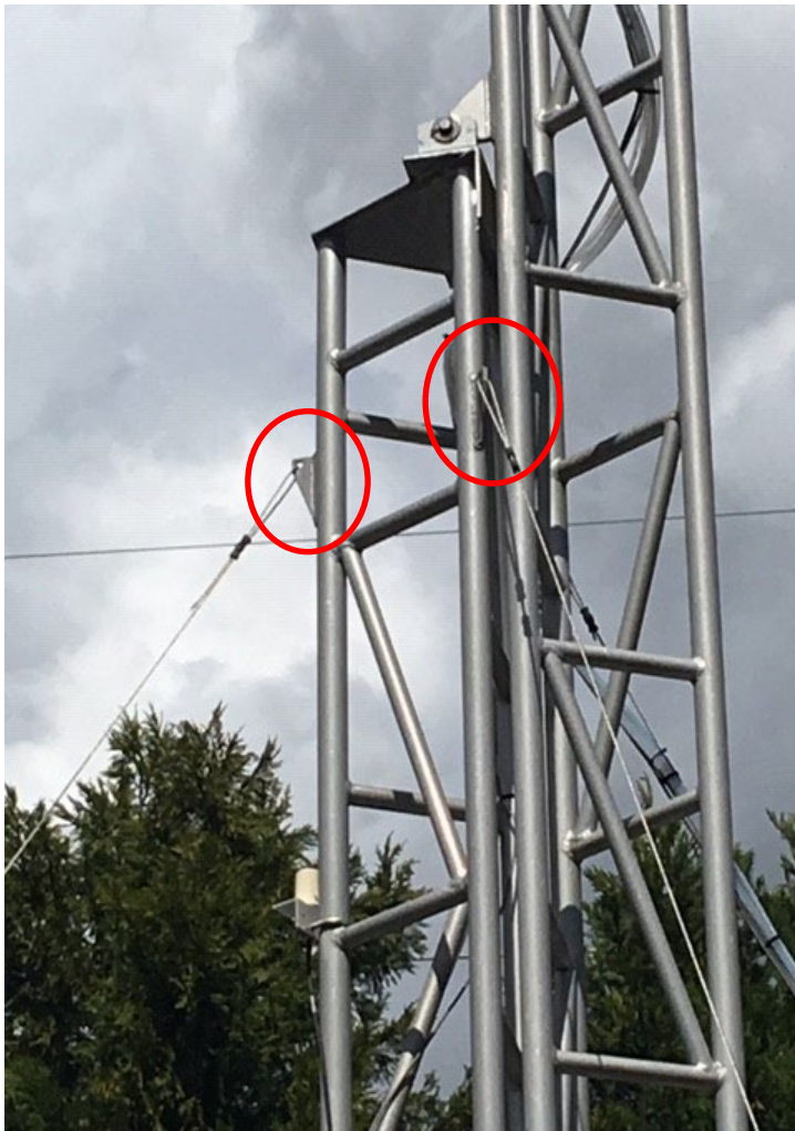
Figure 1. Tower guy wire attachment points (2 of 3 attachment points)
