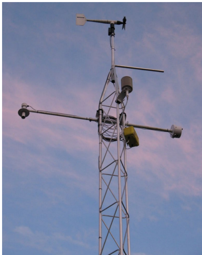
Figure 1. R.M. Young Meteorological System: (from top to bottom) Meteorological Tower with Wind AQ, Directional Cross-Arm, Gill Aspirated Shield for RH Probe, 9-m Aspirated Temperature Sensor Shield and Waterproof RH Circuit Card "Otter" box.
