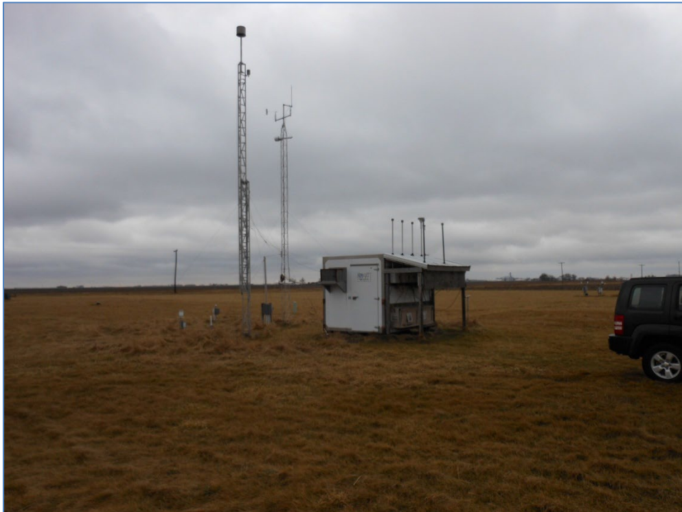
Figure 3. BVL130 CASTNET Sampling Towers and Old Shelter
