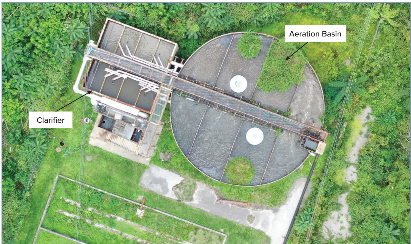
Figure 4. Benham WWTP. Photo by Wesley Turner, KY EEC.
