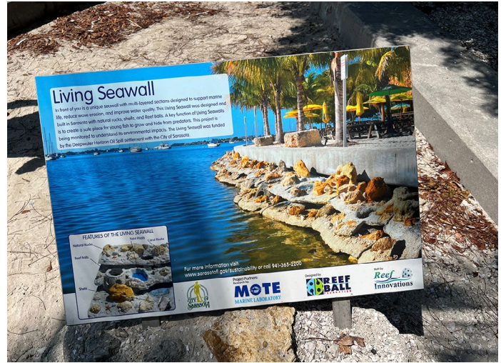
Living seawall signage at Bayfront Park, a demonstration of strengthening existing seawalls with shells, rocks and hollow artificial reef structures during the Sarasota Estuary Program PE site visit.
