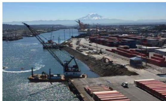
PHOTO: PORT OF TACOMA DOCK REPAIR
