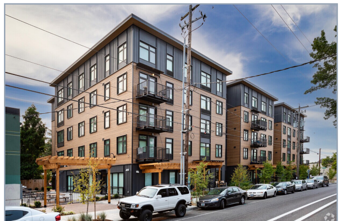
Affordable Housing Apartments in Portland.
