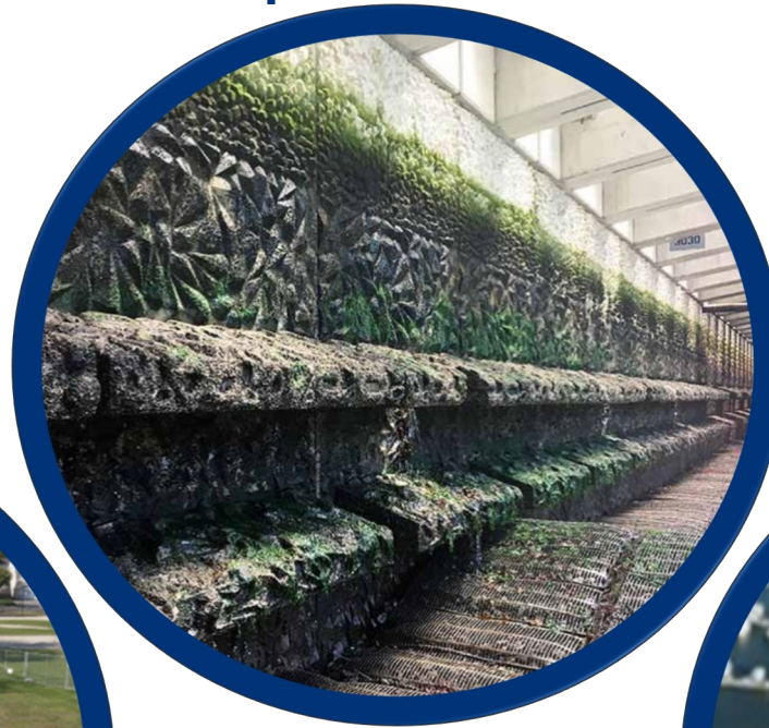
Retrofitted shoreline protection structures
