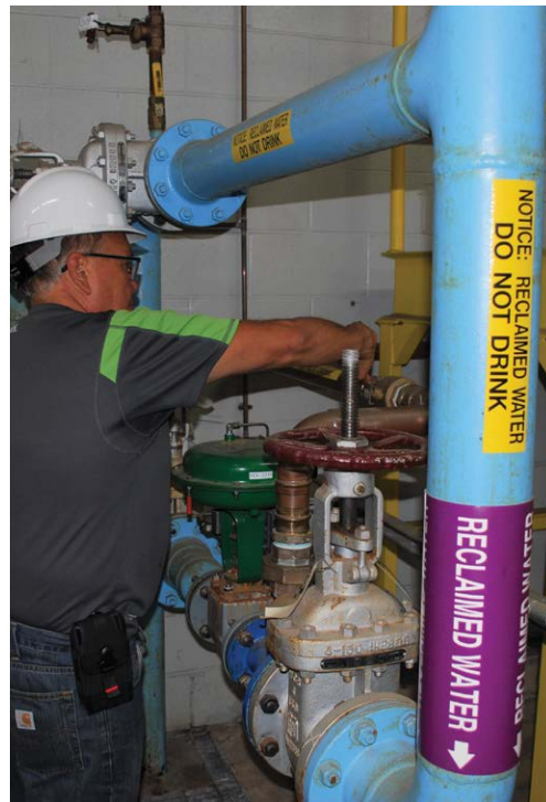
UMass Amherst in Massachusetts offsets its water consumption by using reclaimed water from the Amherst Wastewater Treatment Plant for non-potable applications such as steam and hot water, cooling water, and irrigation.
