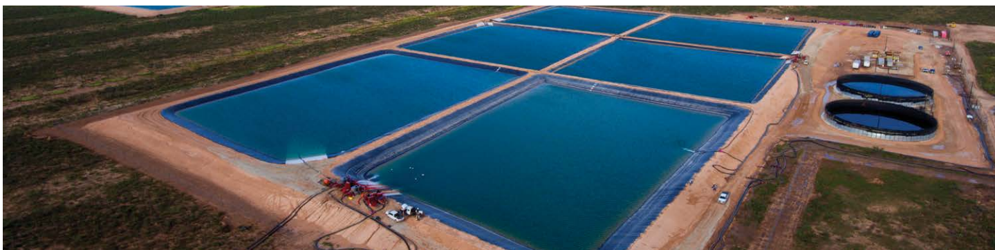
Apache Corporation, an oil and gas company, recycles produced water, reducing its freshwater withdrawals to only 1 to 2 percent. Pictured here is an Apache Corporation facility in Texas.
