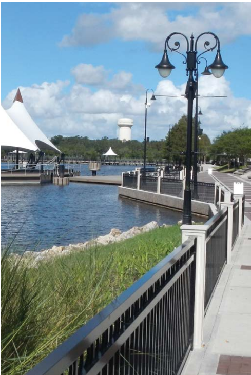
Runoff from a Florida interstate and adjacent drainage basins flows into a regional stormwater facility that delivers reclaimed water to the city of Altamonte Springs for lawn, landscape, and other non-drinking purposes.
