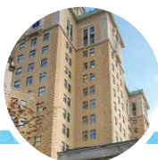
The Hart-Dole-Inouye Federal Center (MI) sends rainwater to a 125,000-gallon cistern, treats and filters the water, and uses it onsite for cooling tower make-up water and irrigation.
