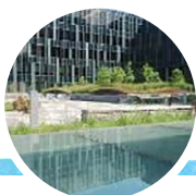
The green roof at the U.S. Coast Guard Headquarters (DC) intercepts, stores, and treats stormwater—up to and including water from a 95th percentile storm—and uses it for onsite irrigation and water features.
