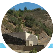
The Santa Rosa Regional Water Reuse System (CA) pumps tertiary treated wastewater 40 miles uphill to steam fields where it generates electricity for 100,000 households as part of the Geysers Recharge Project.
