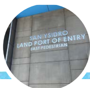
The San Ysidro Land Port of Entry (CA) features a membrane bio-reactor blackwater onsite treatment system, producing non-potable treated graywater that is combined with rainwater for flushing toilets, irrigation, and cooling towers.
