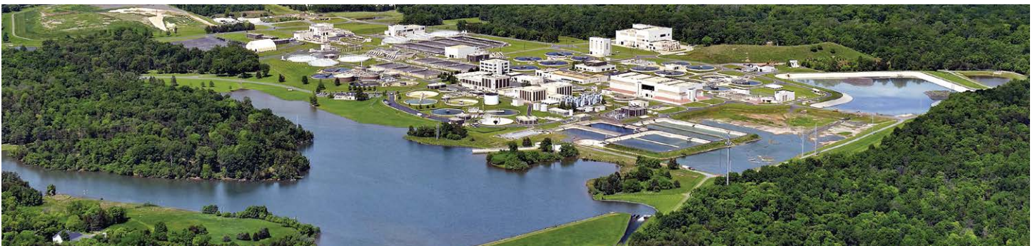
The Upper Occoquan Sewage Authority in Virginia treats wastewater for recharge to the Occoquan Reservoir. Currently about 50 MGD of treated wastewater is recycled, which, depending on hydrologic conditions, is 10 to 90 percent of the drinking water reservoir inflow.
