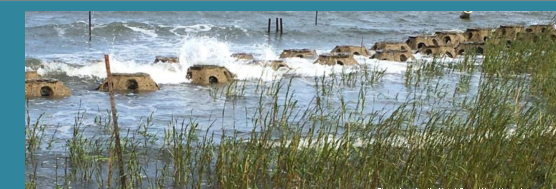
Figure 5. Reef balls promoting marsh growth at Stratford Point, CT.
