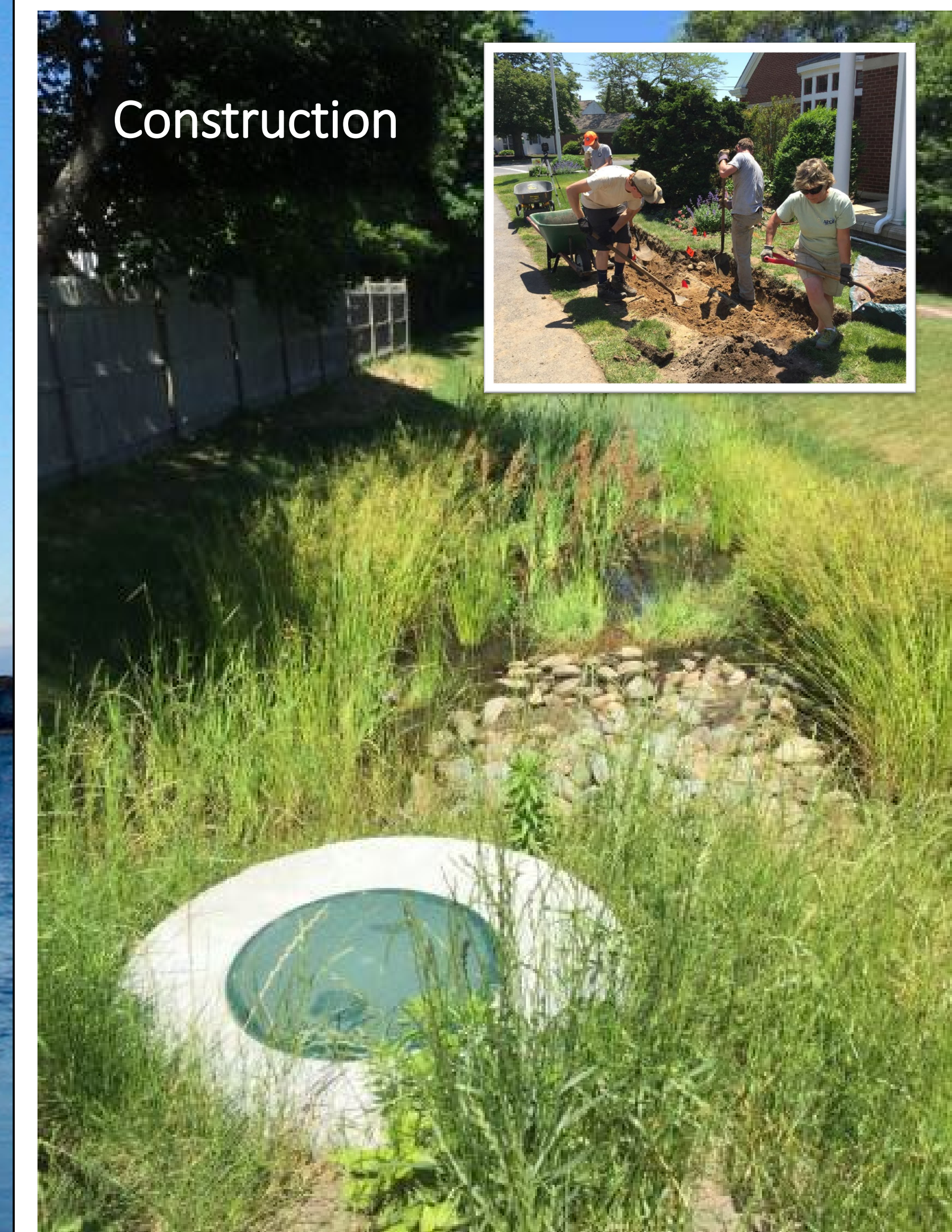
Fall 2018: Construction of 4 BMPs Spring 2020: Construction of minimum 2 additional BMPs
