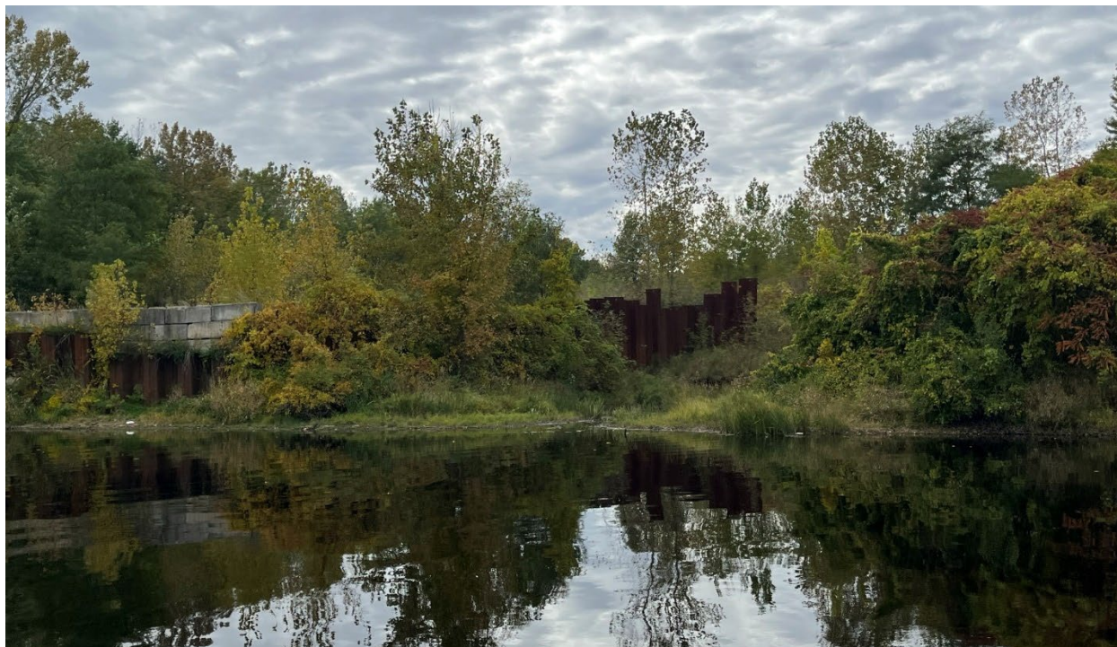
Photo 5. NYSDEC Moreau launch and loading area during dredging (Reach 8).
