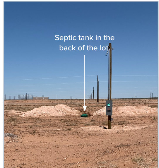
Figure 3. Septic tank constructed for new lot.
