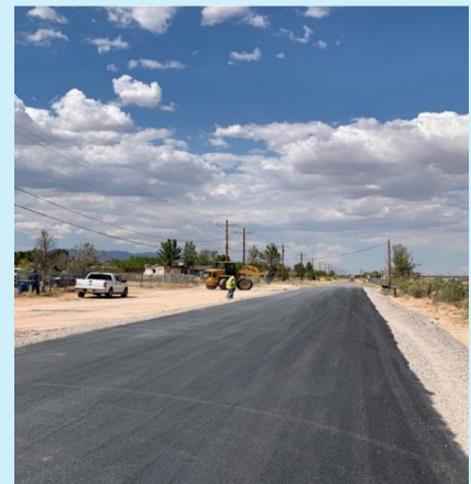
Figure 1. Construction activities on Edna Street, Chaparral, New Mexico.
