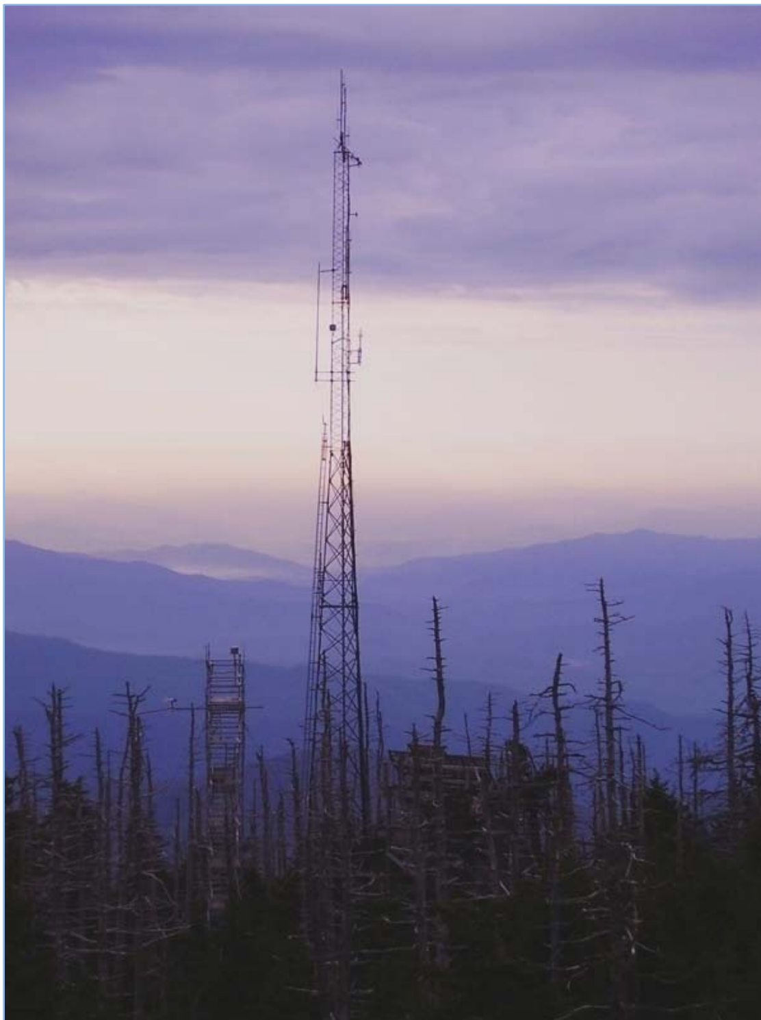
View of the Cloud Collection Tower and NPS Radio Tower
