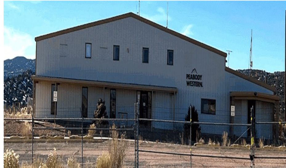
N-8 Operations Building
