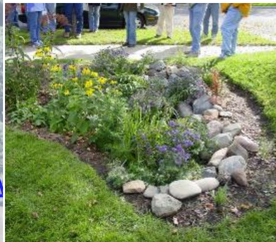
Rain Garden for Stormwater Runoff
