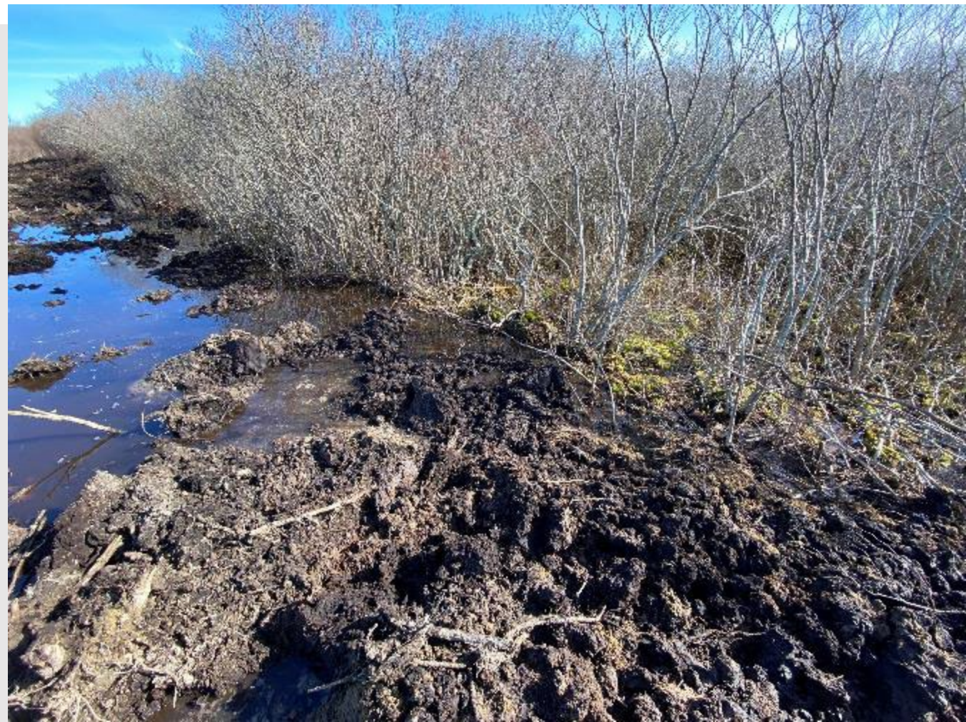
REMOVING BERMS/ RECONNECTING BVW
