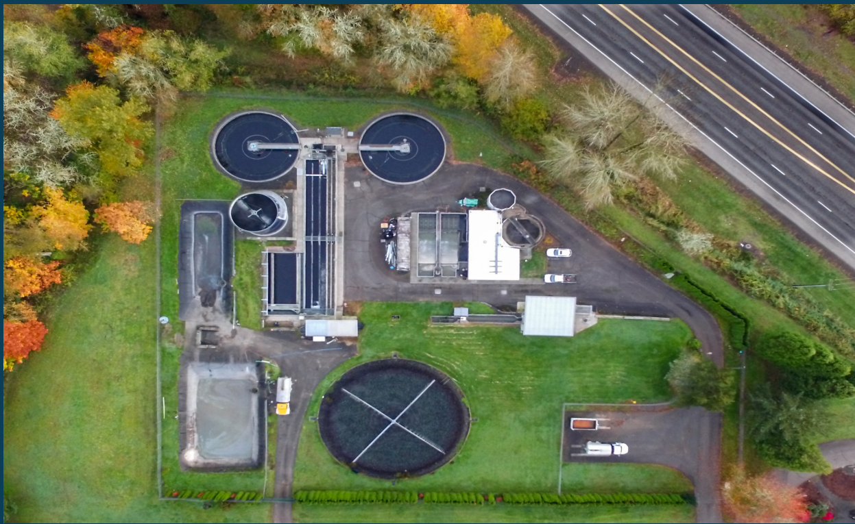
Aerial view of current wastewater treatment plant
