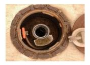
**SPILL PREVENTION WITH SPILL BUCKETS.** Spill buckets attached to USTs temporarily contain small product spills during delivery. However, improper spill bucket maintenance could lead to soil and groundwater contamination. Follow these tips to keep your spill buckets in good working order and to reduce risks.
