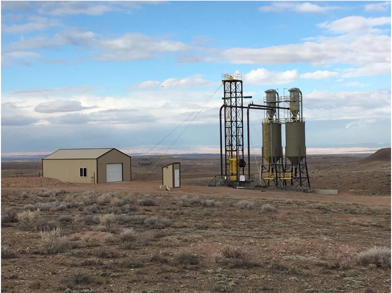
Figure 5. Surface photo of TRM#1 mine (future site of Outfall 001)
