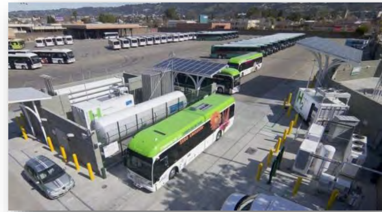
AC Transit – Emeryville On site H2 production (Electrolyser)
