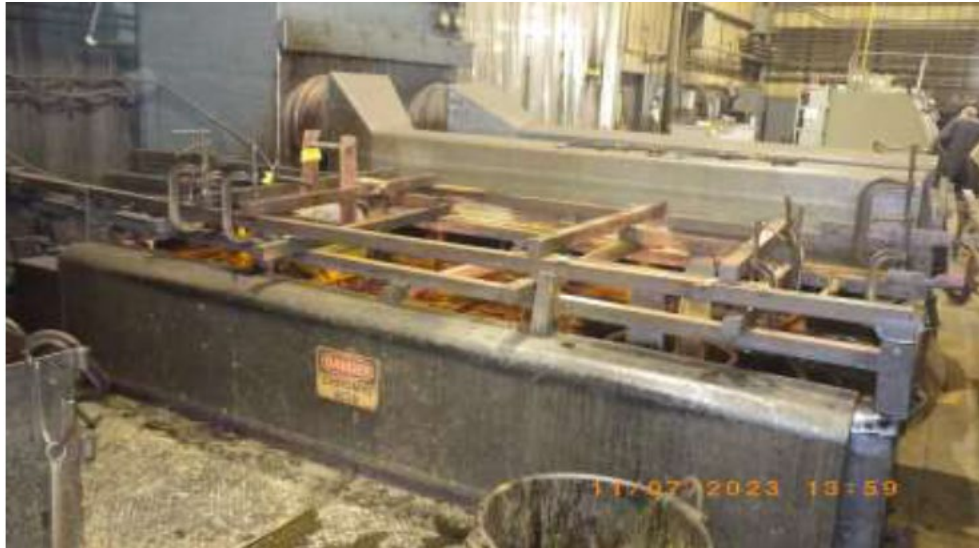
Figure 6 - Chrome Plating Tanks A and B
