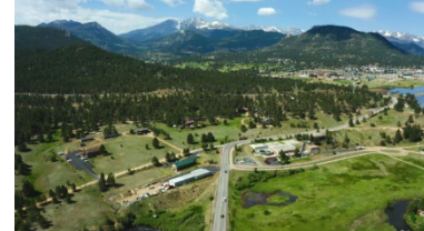
Photo credit: Upper Thompson Sanitation District
