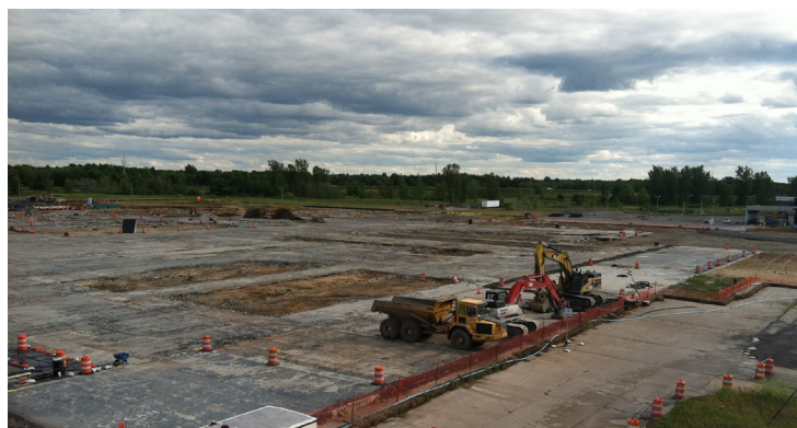
Slab demolition at the GM Massena site.
