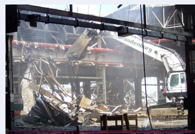
Demolition of the former GM manufacturing building, July 2011.
