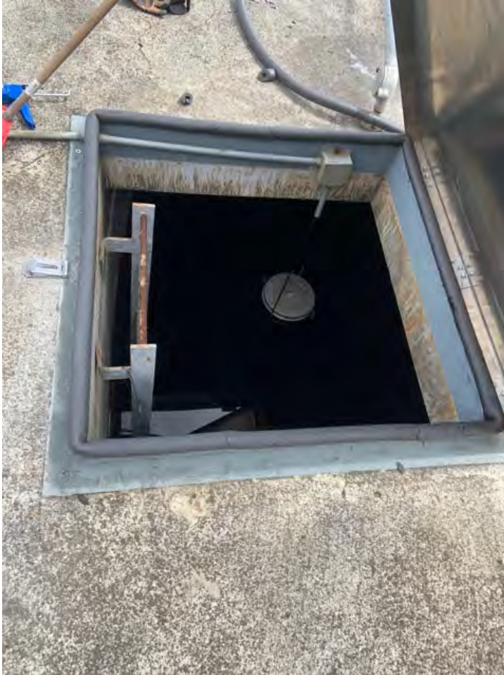
New tank hatch with gasket
